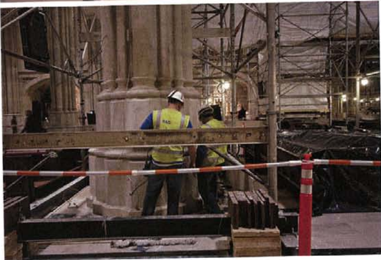
Workers cluster around a column.
